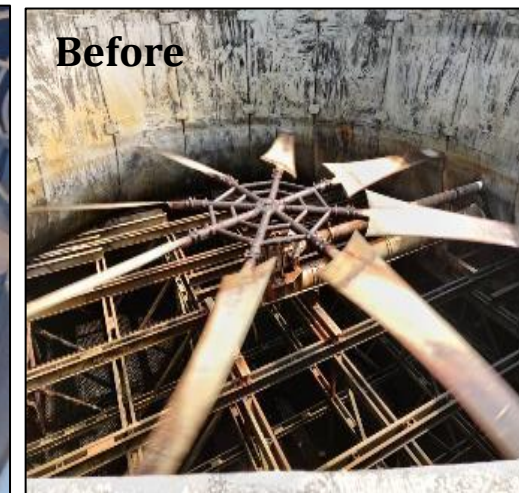
Replacement of CT Fan blades with redesigned blades
