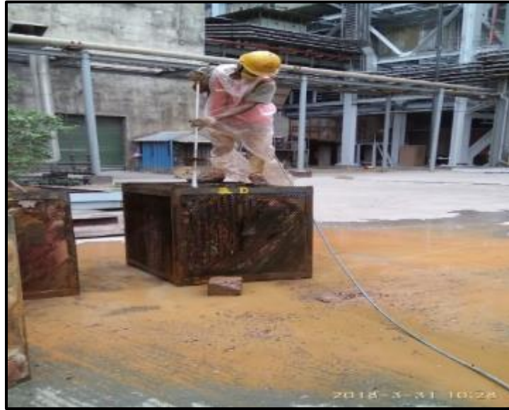
High pressure water jet cleaning of basket APH Basket Replacement
