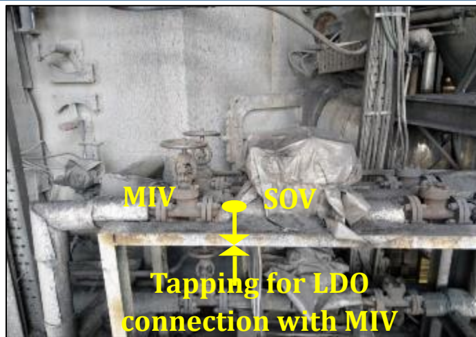
Elimination of HFO guns with LDO guns
