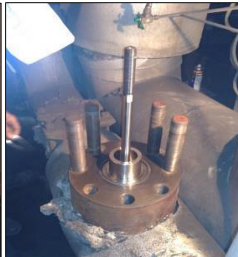
Upgradation of BFP RC valve trim set from single stage to multistage
